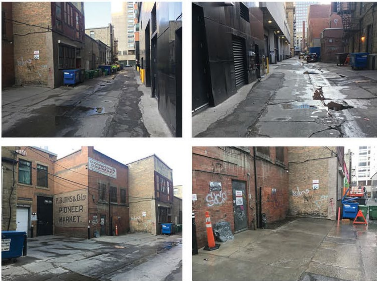
Figure 15. GAP, 8 ave, SW alley location condition.
