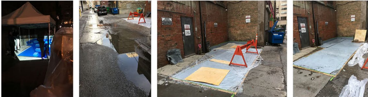
Figure 25. First-night painting attempt during rainstorm and next morning results. Plastic sheets were used to cover the initially completed undercoat (gray painted areas).
