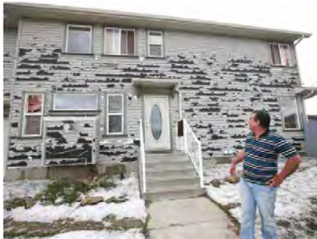
Hailstorm Damage
