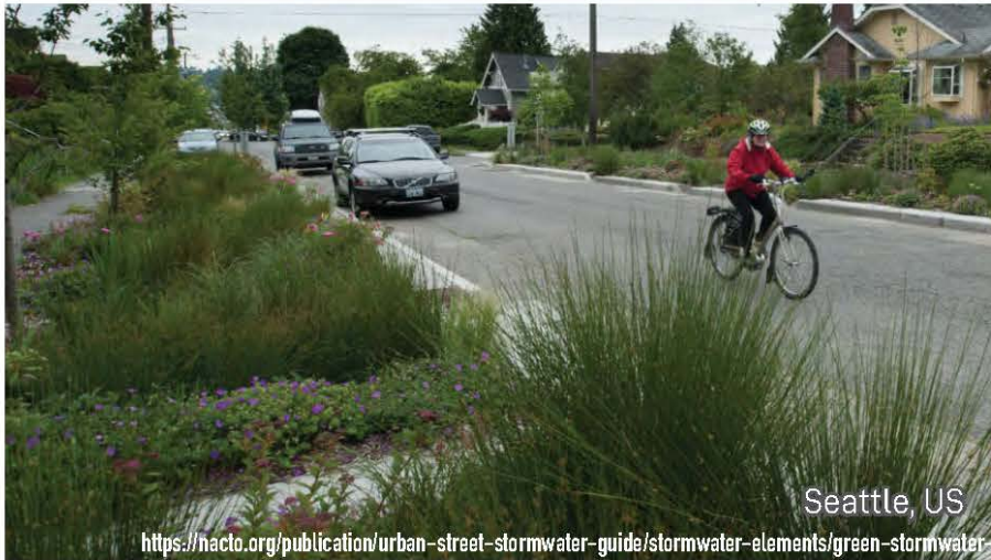
Bioretention Swale
