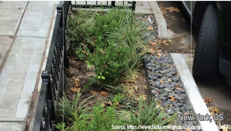
Walled Bioretention Planter
