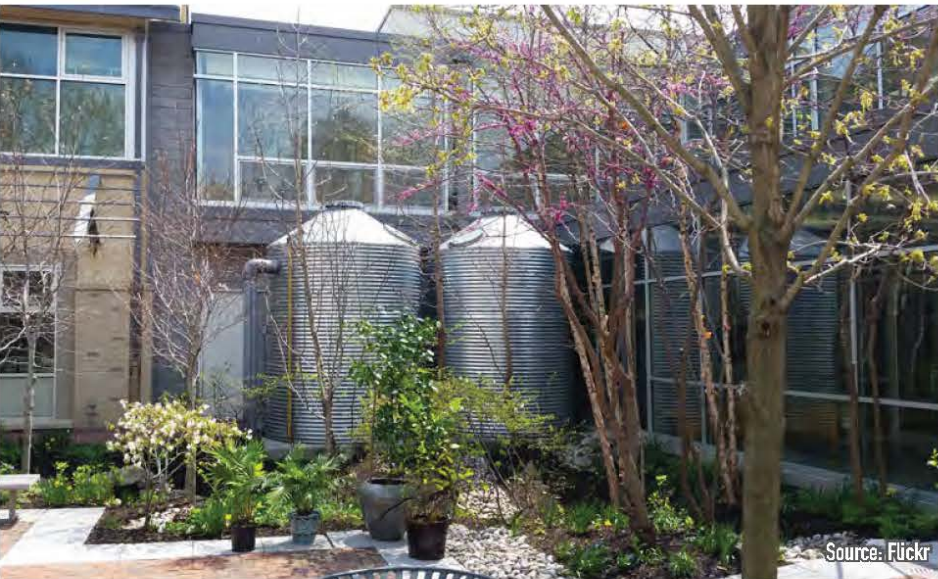
Commercial Rainwater Harvesting
