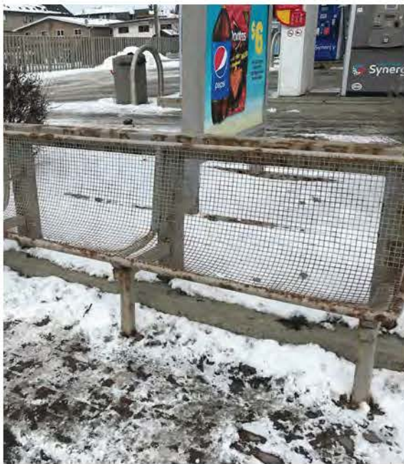
Long periods of cold and wet climate creates rust and degradation of infrastructure
