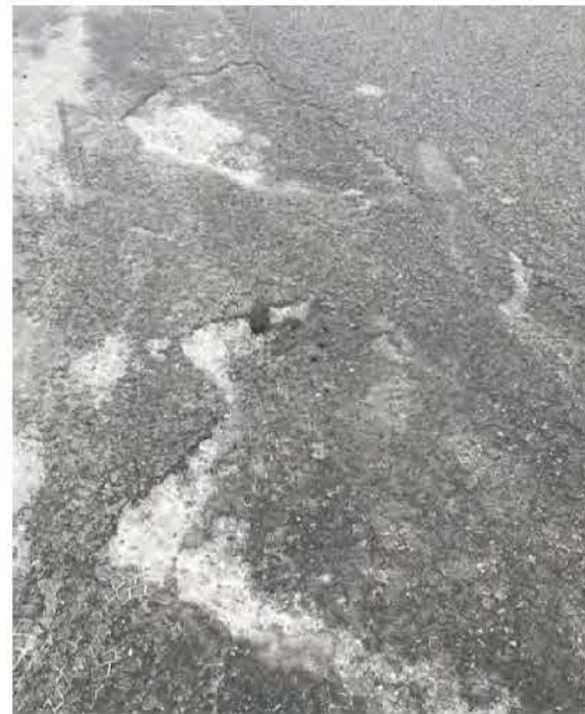
Asphalt becomes broken down from salt and gravel build up in Winter. This creates dangerous walking conditions.
