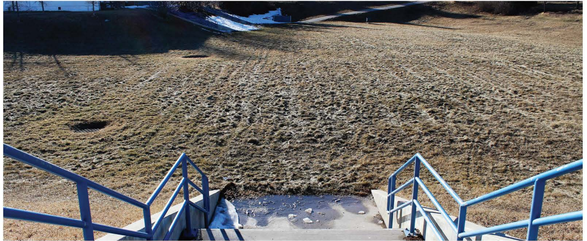
View of current storm water catchment area from the east to west
