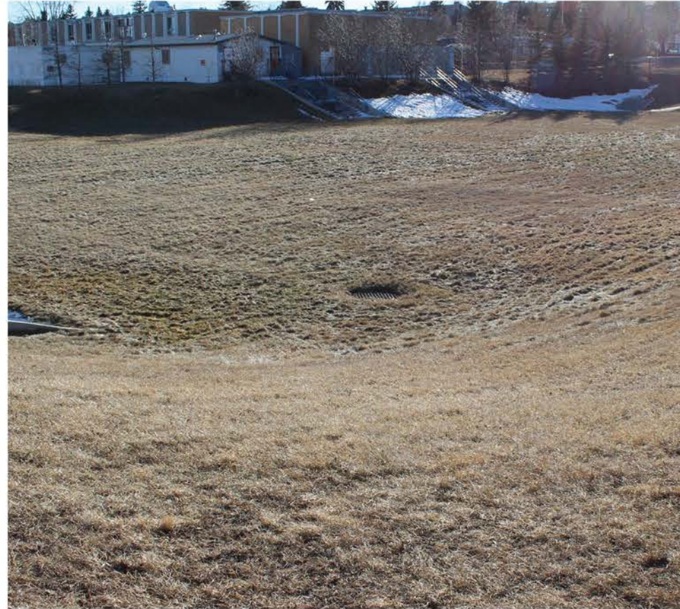
Existing conditions of drainage pond on Haddon Road
