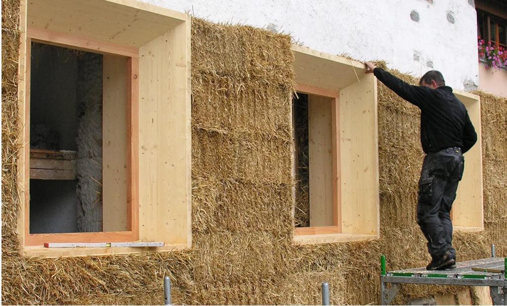
Casa Steila Mar deep energy renovation, Atelier Werner Schmidt, Switzerland, 2014.
